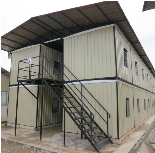
Foto 5 : CLQ Tanjung Bin Power Plant, Pontian, Johor
